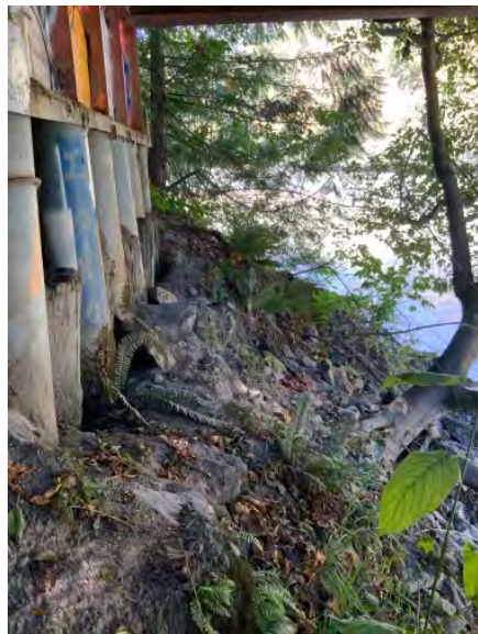
Right Bank Abutment when facing downstream
