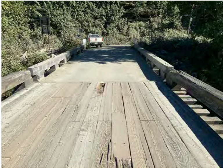
Approach from Left Bank when facing downstream
