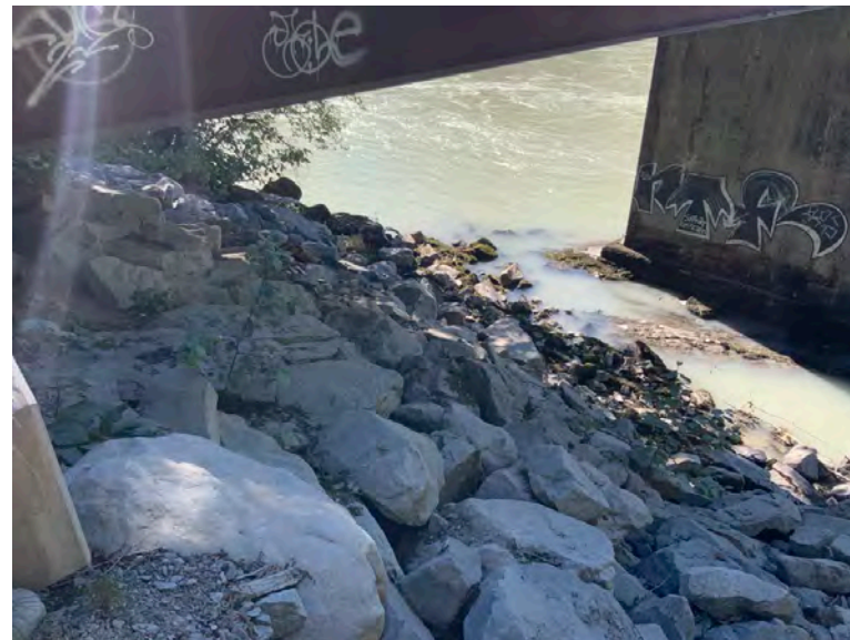
Left Bank Abutment when facing downstream
